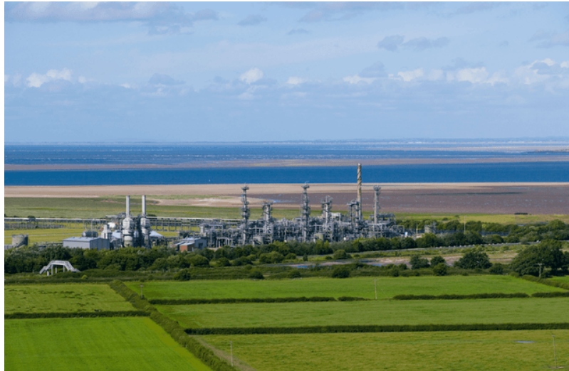
Point of Ayr Terminal
